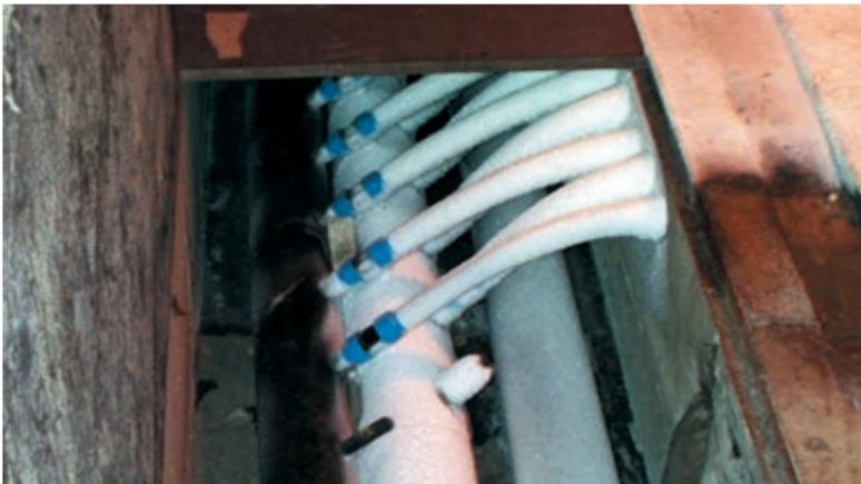
Plastic rink piping connections to the distribution and the collection mains (thermally insulated).
